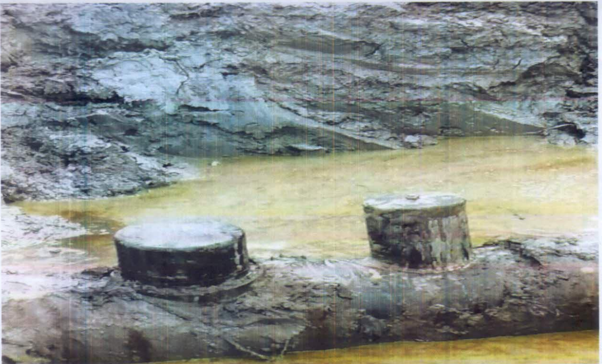
PICTURE SHOWING AFTER REPAIRS OF THE SPILLED POINT.
